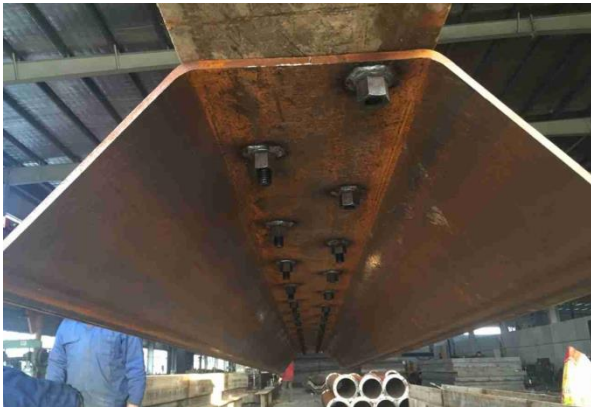
图8 螺栓连接施工 Fig. 8 Bolted construction
