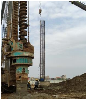
图3 双动力头套管钻孔 Fig. 3 Double power head casing drilling
