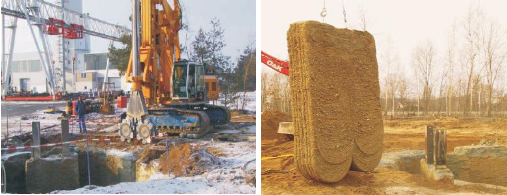
(a) CSM工具 (2004, Bauer/Bachy Soletanche)
