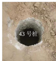
Fig. 1 Construction sequence of CFG pile and concrete surface sinking at the top of pile 43
