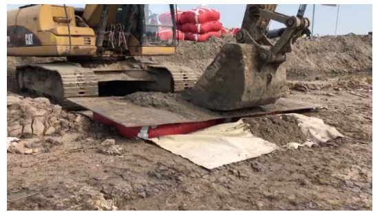
图 6 地固件作为临时道路 Fig. 6 Ground improvement unit as temporary road
